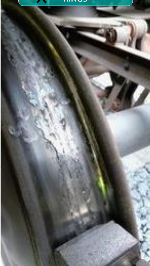
HEAVILY WORN BEARING RINGS ✗ RINGS
